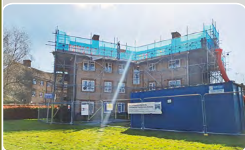
A new roof being installed at Godwin Court in Horsham.
